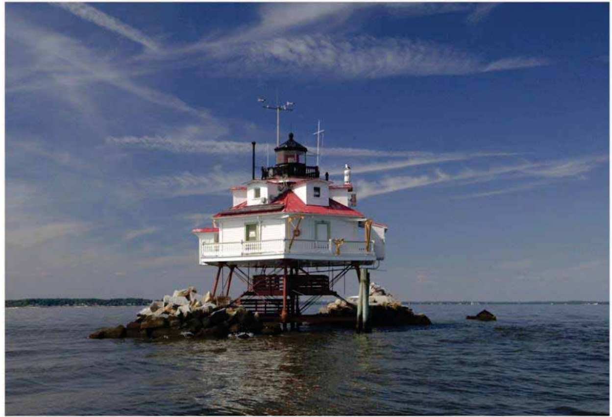
THOMAS POINT SHOAL LIGHTHOUSE CHESAPEAKE BAY
